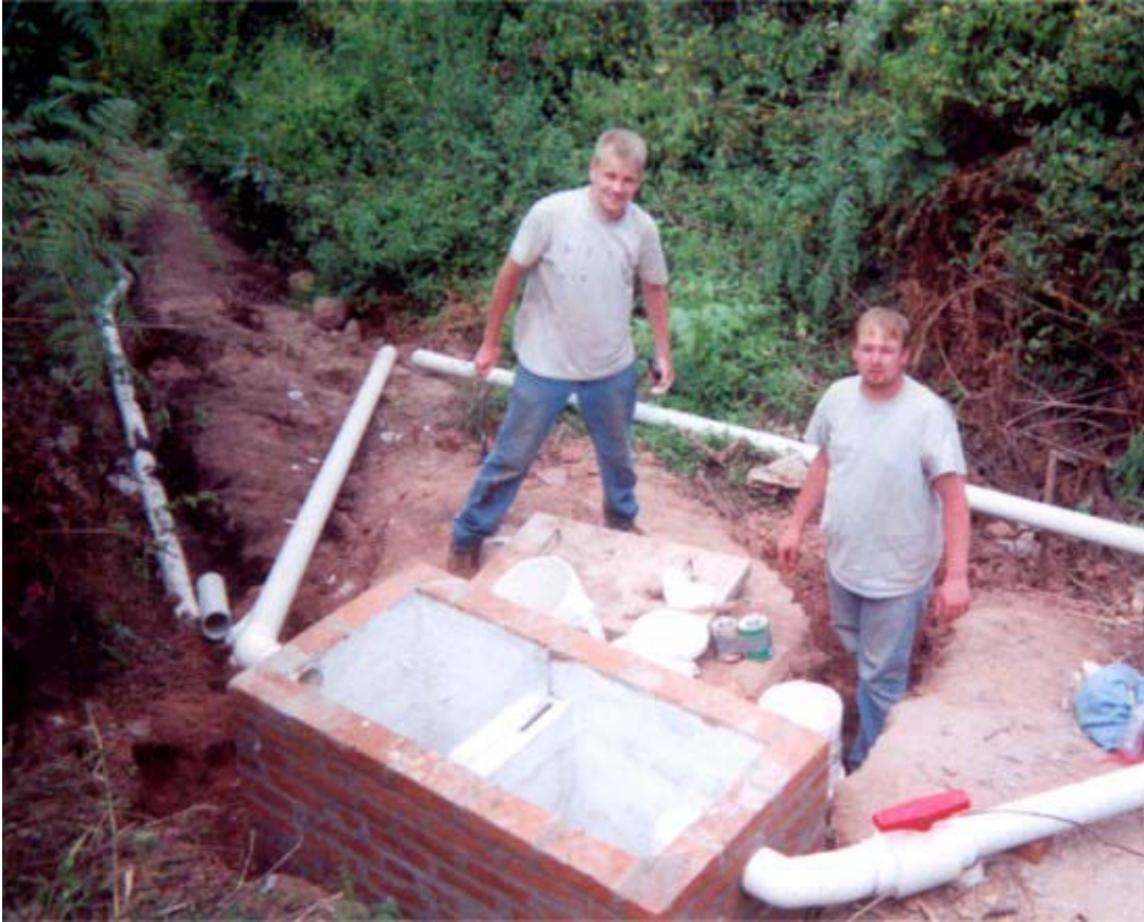
Figure 2: Dordt Students Installing a Crop Irrigation System in Honduras
